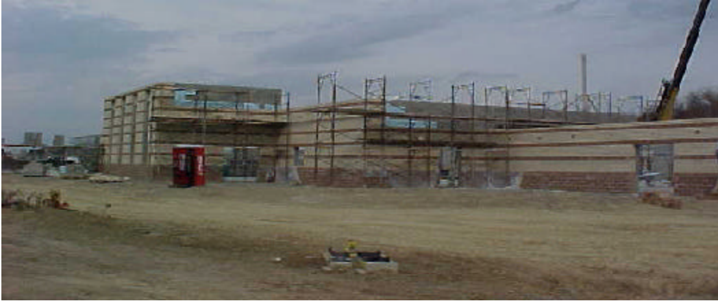
The New STO-ROX Middle School under construction
